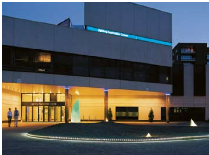
Philips Lighting Application Center Eindhoven, Paesi Bassi
