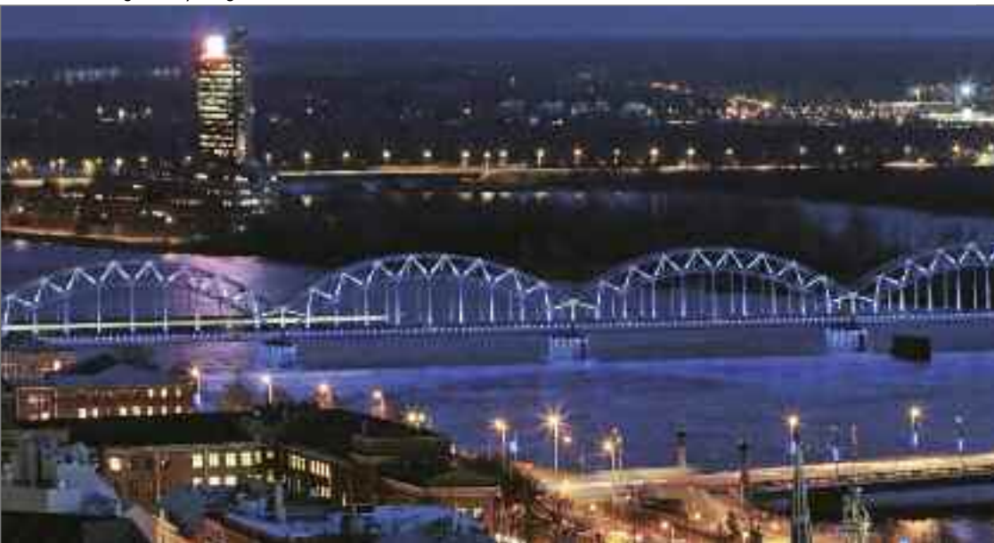
Letonnie - Riga Railway Bridge
