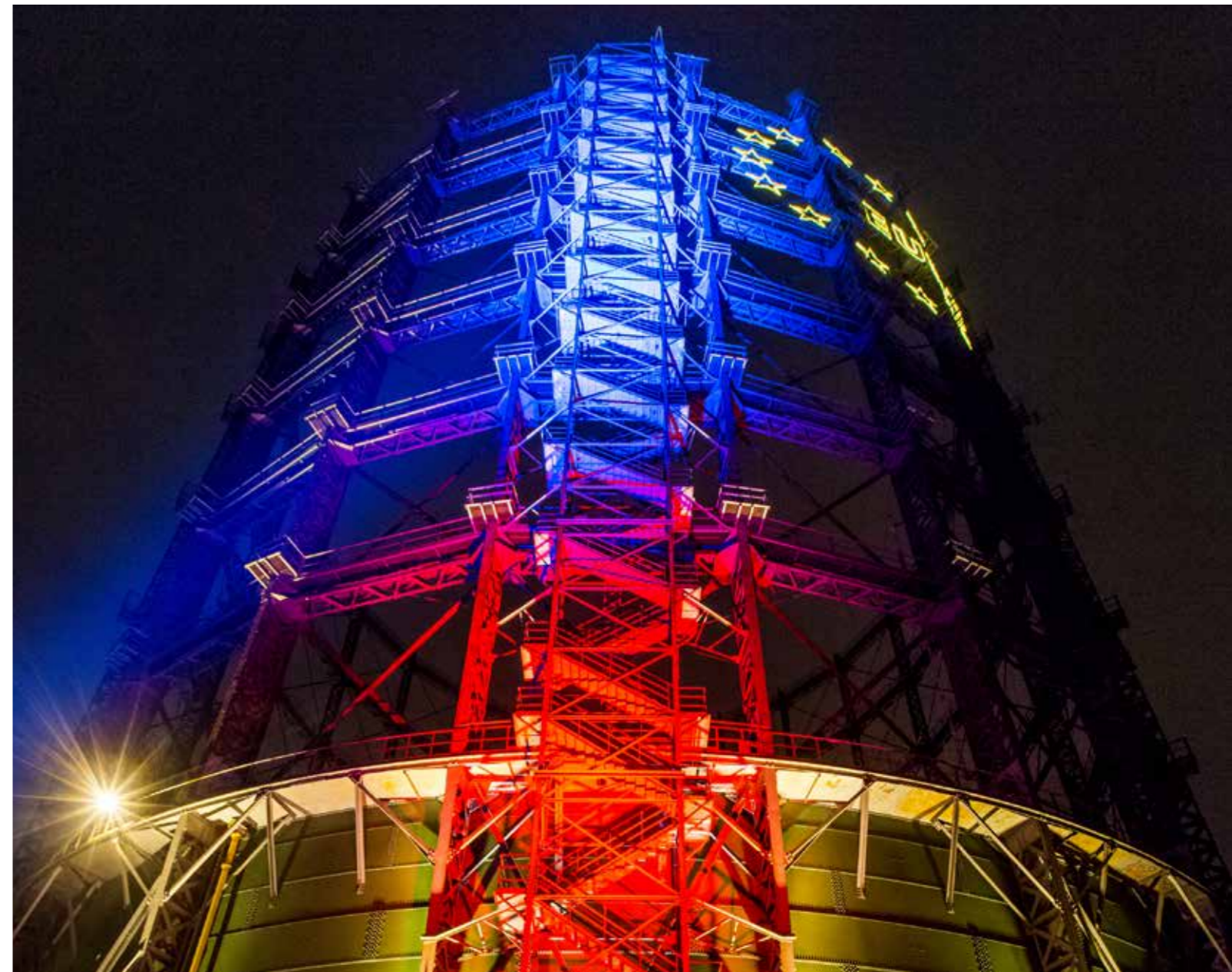
Lighting concept installation
