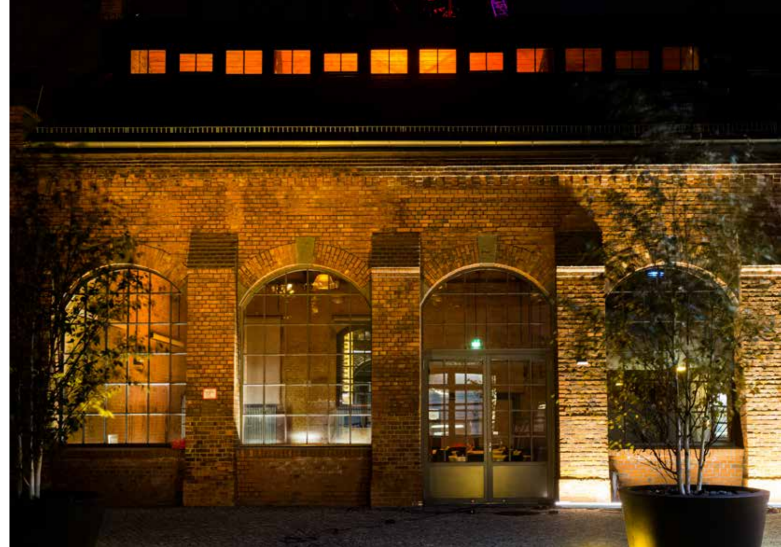
Lighting concept installation
